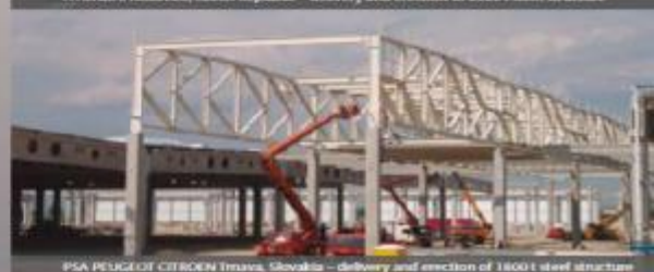
PSA PEUGEOT CITROEN Trucks, Slovakia - delivery and erection of 1800 t steel structure
