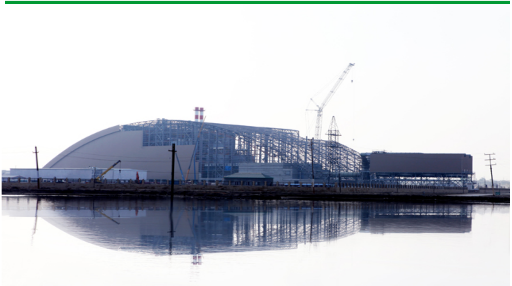
The construction of the plant in 2011
