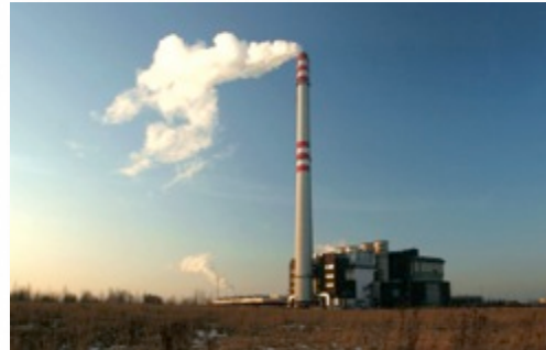
PRIORITY of energetical use of waste – WTEP Malešice
